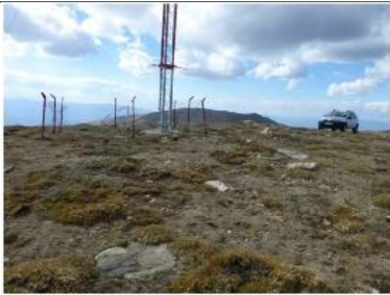
Figure 24: Project area setting of the planned Turbine 17 location
