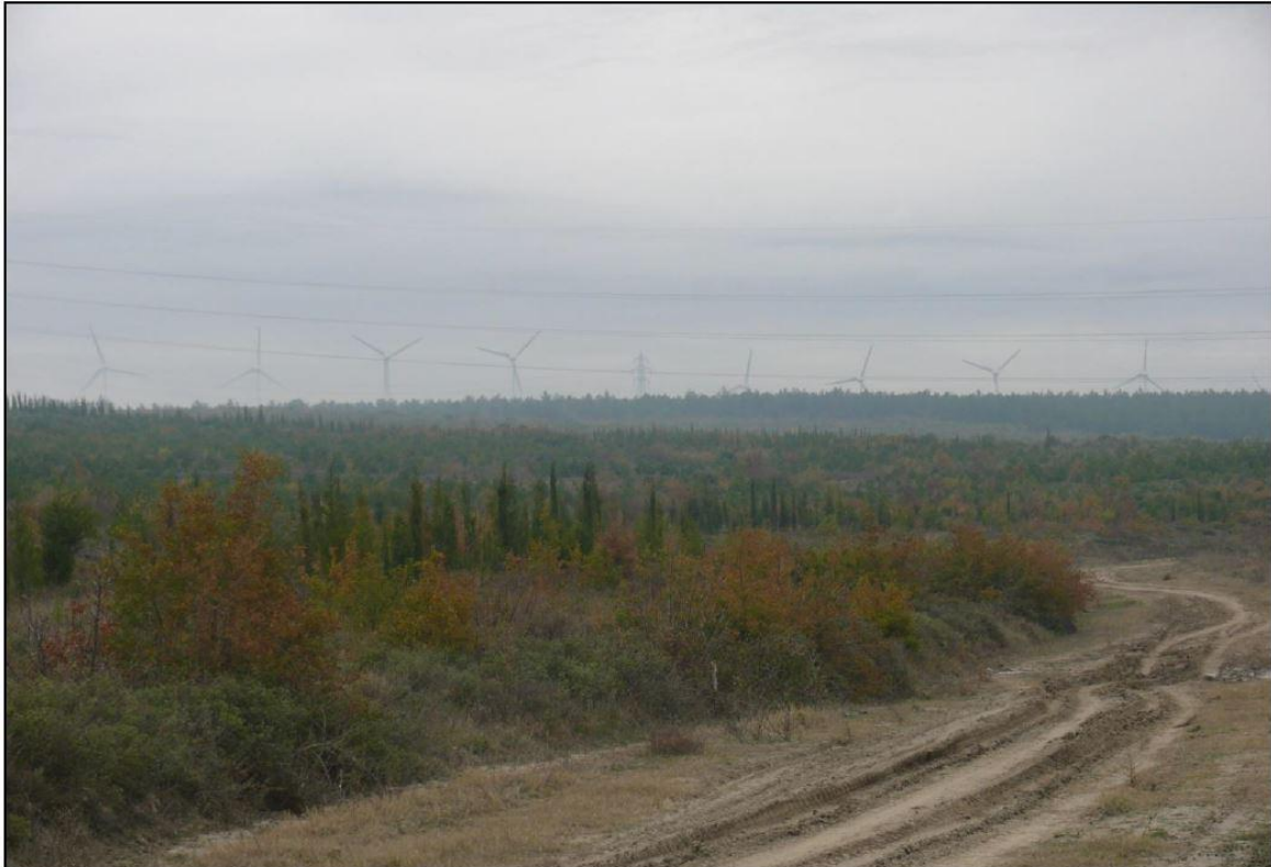
Figure 11: Turbines of the İntepe WPP approximately 1.5 km to the north-northwest of the Project Area
