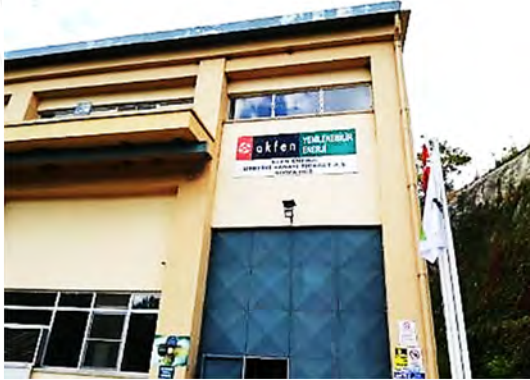
Picture208 SIRMA HEPP POWER PLANT SITE CURRENT SITUATION
