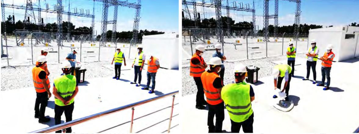
Picture 92 DENİZLİ WEPP LEAKAGE & SPILL DRILL VISUAL_12.06.2020
