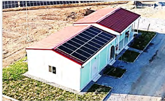
Picture 124 IOTA M. FIRINCI GES Rooftop Photovoltaic Panels
