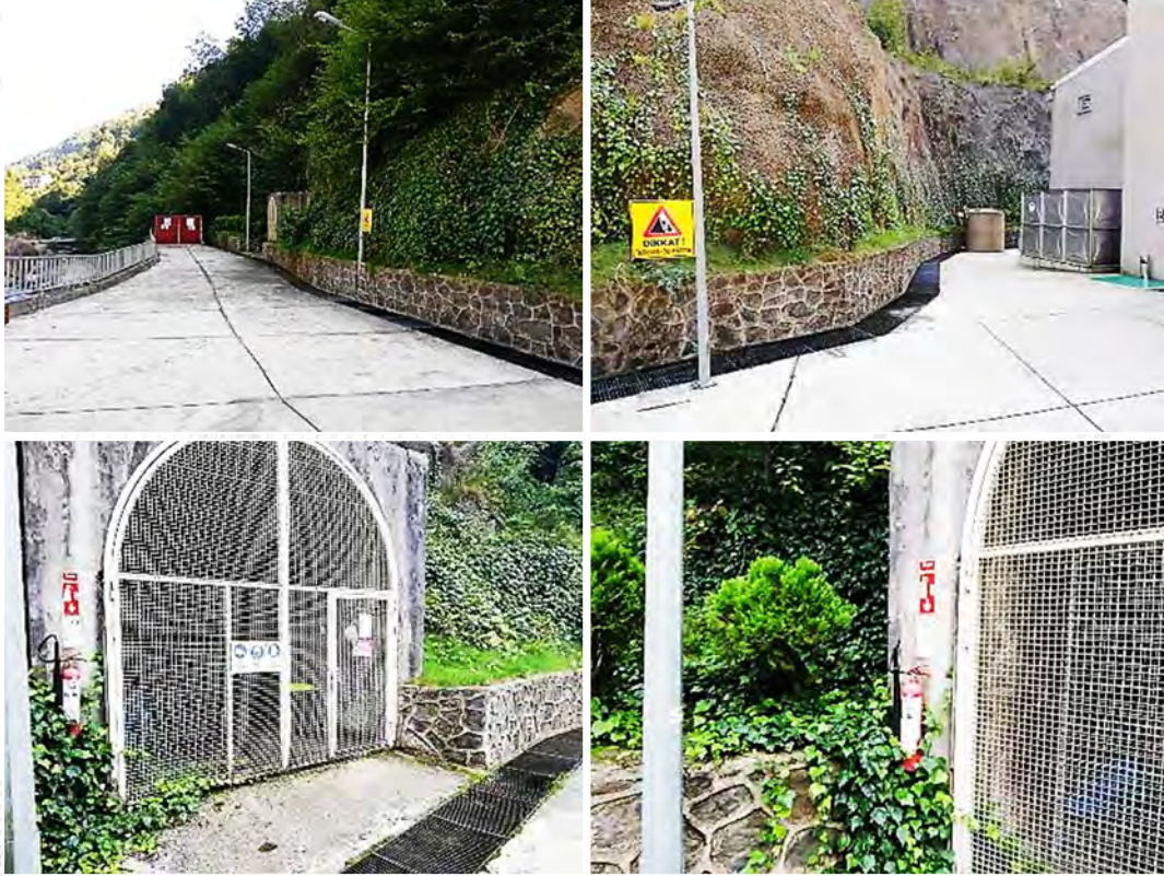
Picture209 YAĞMUR HEPP POWER PLANT SITE CURRENT SITUATION
