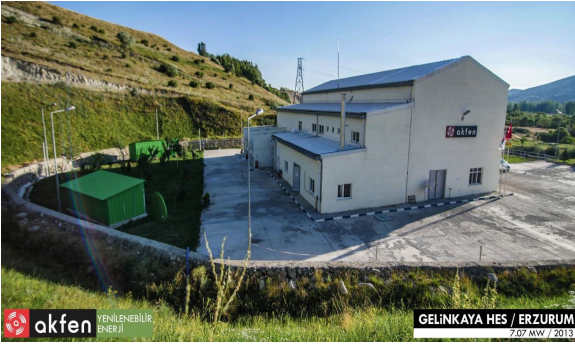
Picture 6. GELİNKAYA HPP PHOTOS
