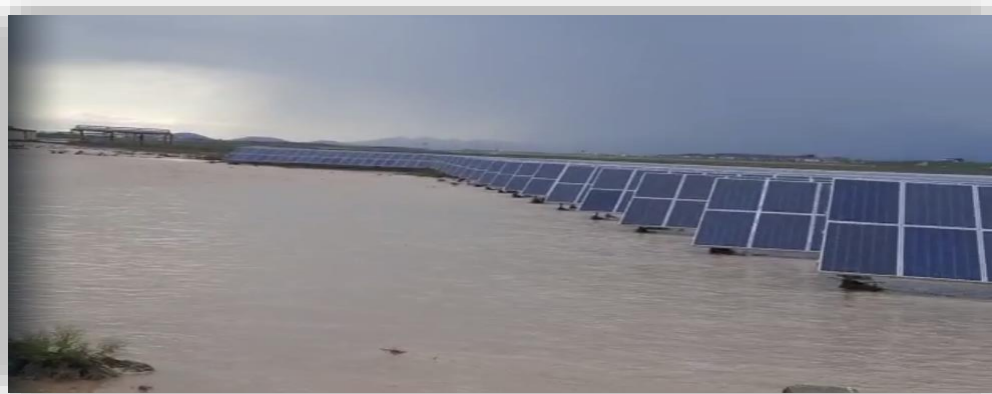
Picture 6. YAYSUN-MT DOĞAL SPP FLOOD PHOTOS
