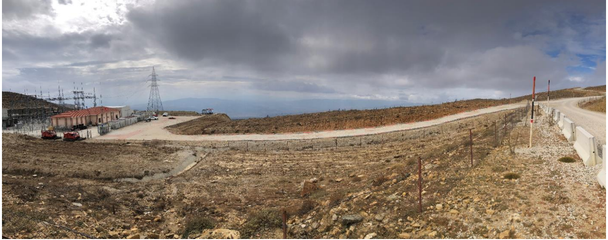
Picture 39. LANDSCAPE AND REHABILITATION WORKS ON DENIZLI WPP SITE
