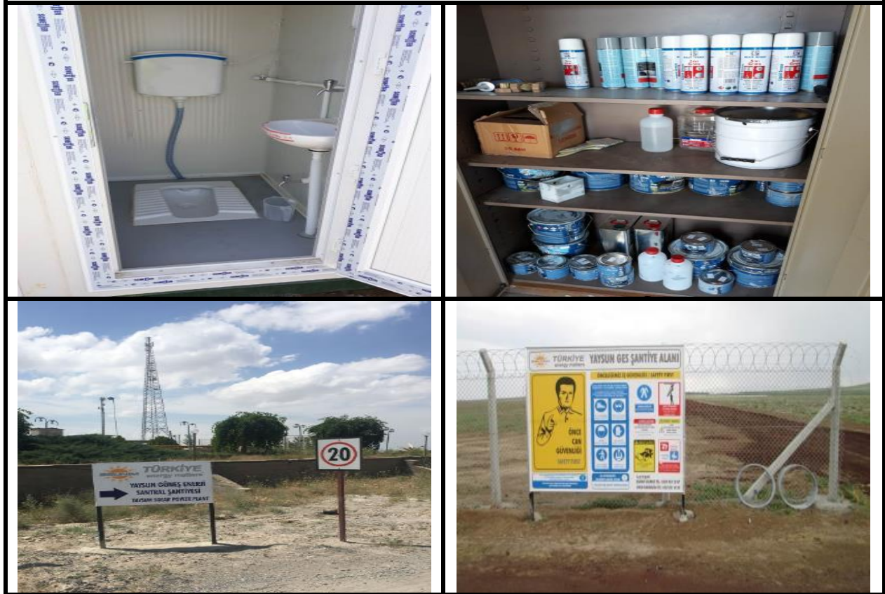
Photograph 19: Examples of OHS Practices at Construction Sites
