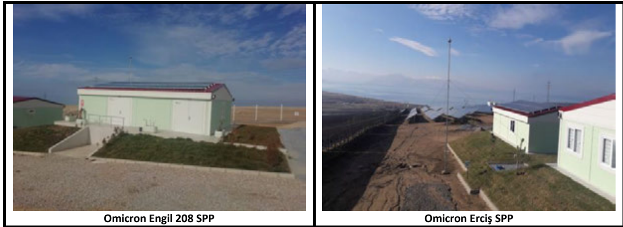
Photograph 22 - SPP Operations Off Grid System
