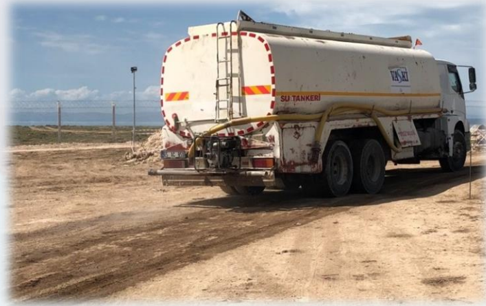
Photograph 95- Image of dust prevention measurement taken at construction site
