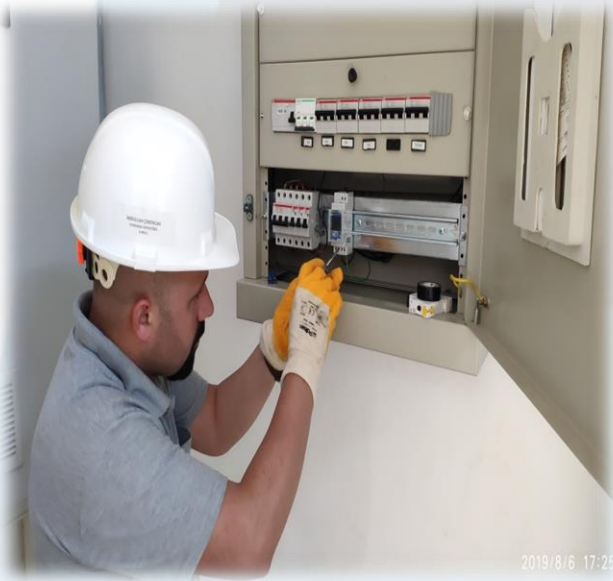
Çamlıca III HEPP-Maintenance of a panel
