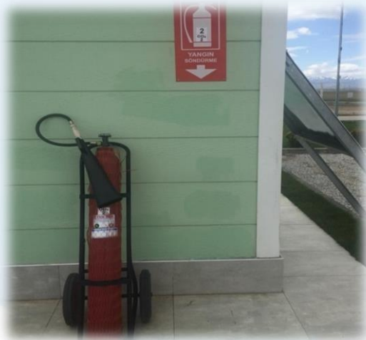
ME-SE SPP-Fire Extinguisher
