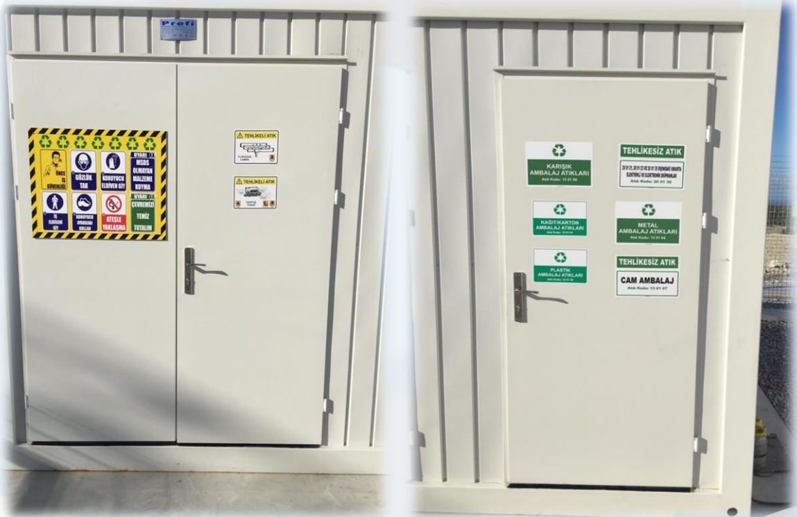
Photograph 89- Hasanoba WPP-Temporary Waste Storage Areas (Hazardous and Non Hazardous Waste)
