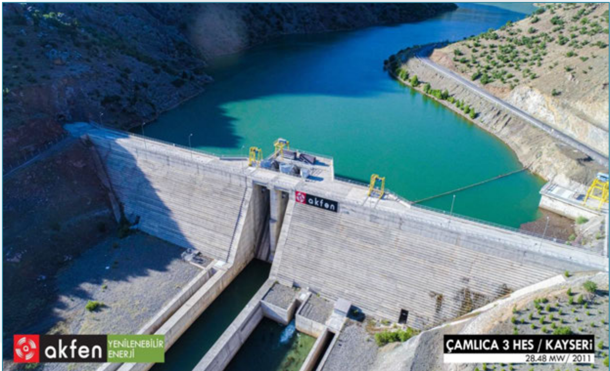
Photograph 5- Çamlıca III HEPP
