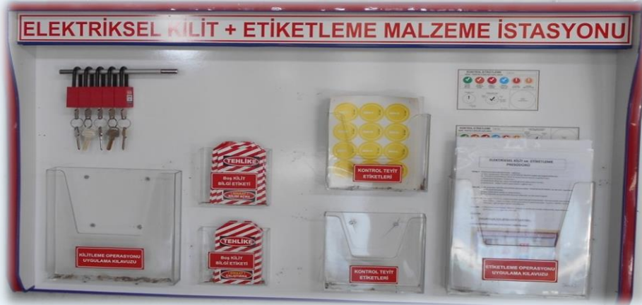
Kavakçalı HEPP-LOTO Station
