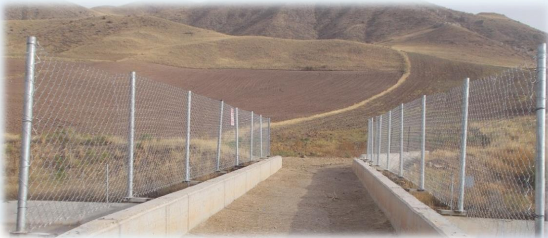
Saraçbendi HEPP Transmission Cannal Fauna Transition Structure
